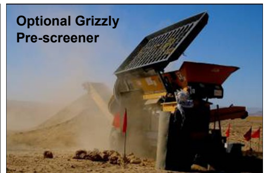
Loading the Hopper for Screening
